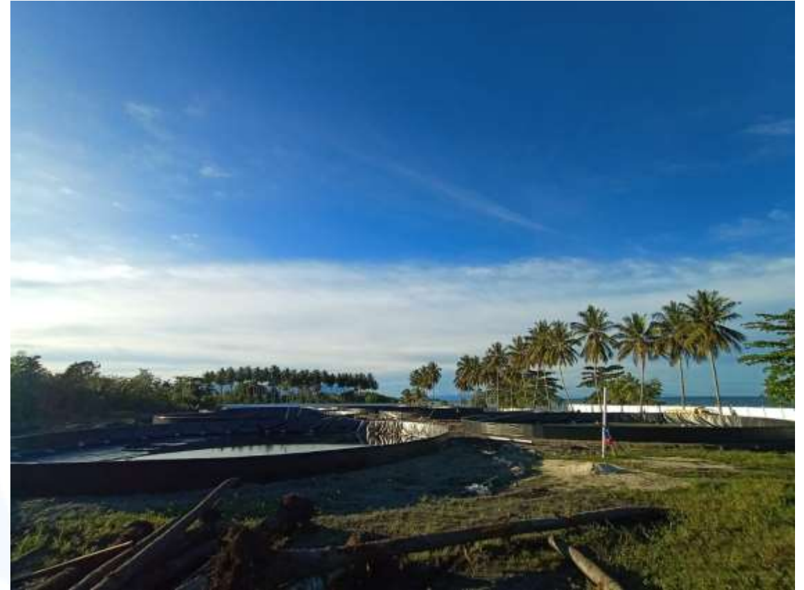
Tambak Udang, Kolam Bulat Geomembrane 0.5mm – 15 kolam Toli-Toli, Sulawesi Tengah
